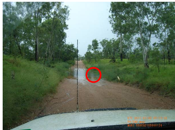
Unknown causeway with significant hole requiring immediate attention.
